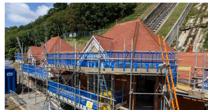
12 months ago the lift looking like a building site, scaffolding has now gone and one step closer to opening
